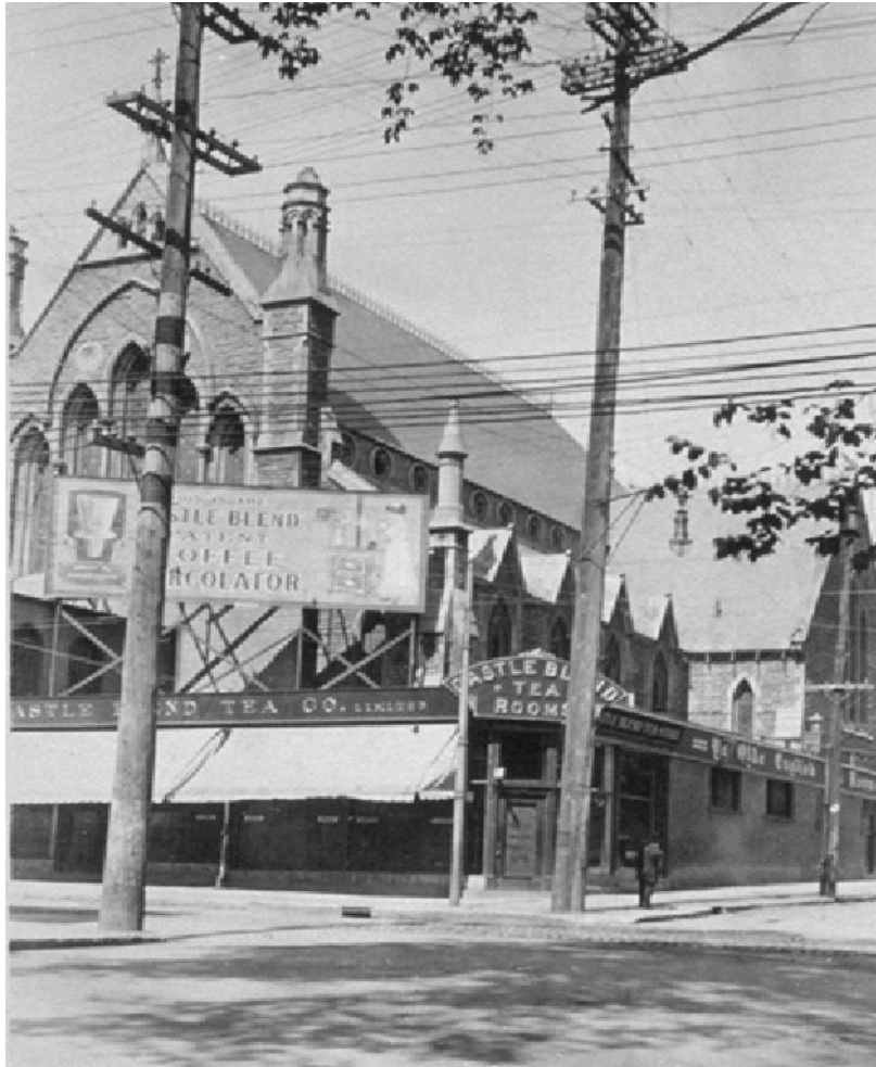
Figure 4: The Original Emmanuel Congregational Church Being Transformed into Shops, 1911 (Bibliothèque Nationale du Québec, Massicotte Collection. The original source of this image is unknown. A similar photograph appears in the Montreal Witness , 16 March 1912).
